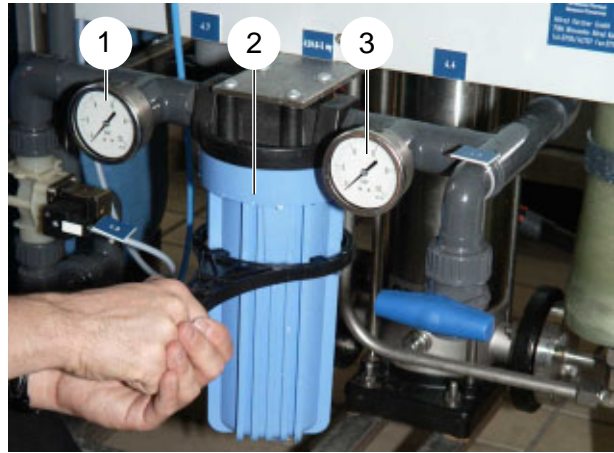
Figure 17 Replacing the fine filter
